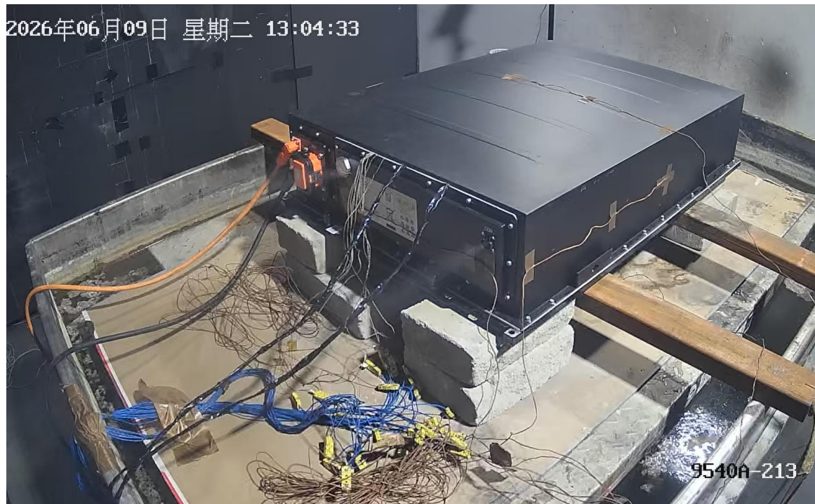
1 st cell thermal runaway induced [13:04]
