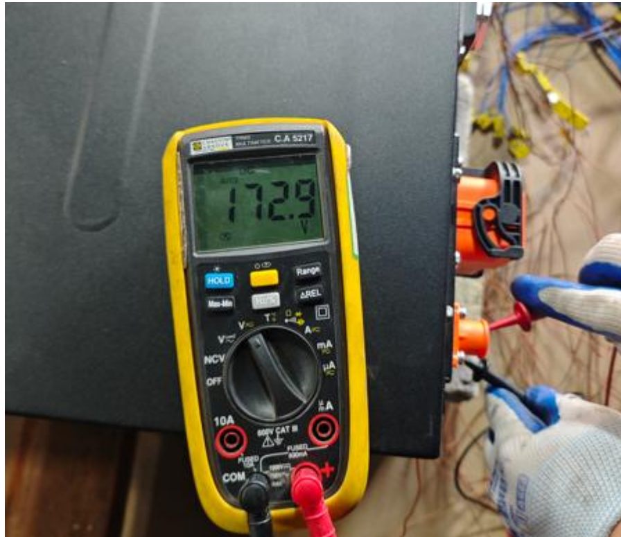
Module voltage after 1h rest [172.9 V]
