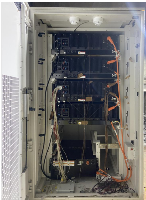
View of Smart String ESS, model: LUNA2000-241-2S1
