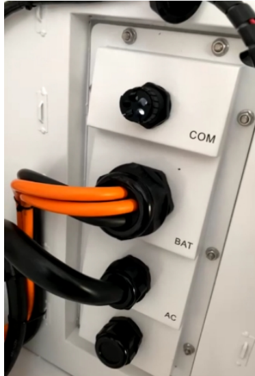
Figure 7- 12 Steps of threading cable
