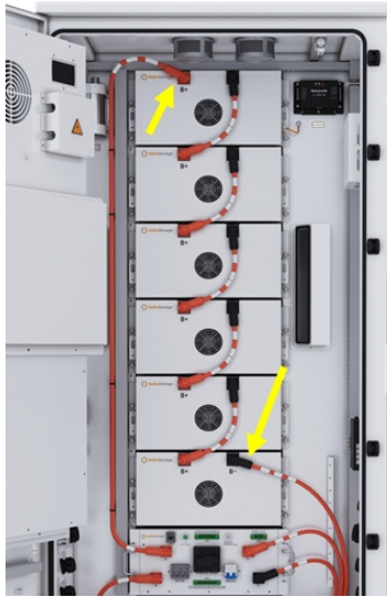
Figure 8-1 Check cable connection
