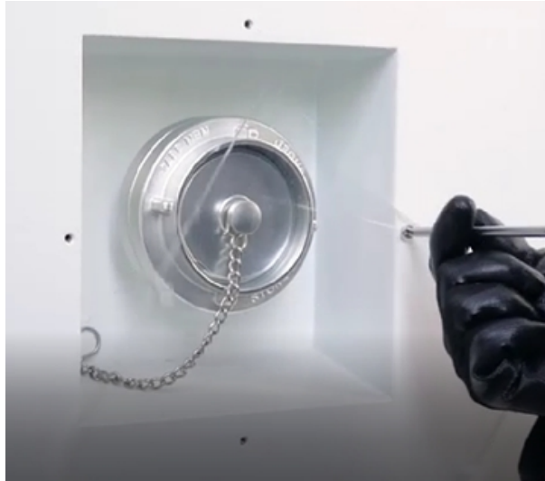
Figure 7-46 Remove the water inlet cover
