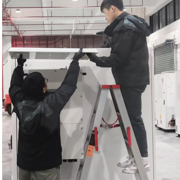
Figure 7-8 fixing the sunshade to cabinet enclosure
