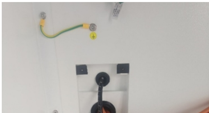
Figure 7-35 Panel ground cable installation
