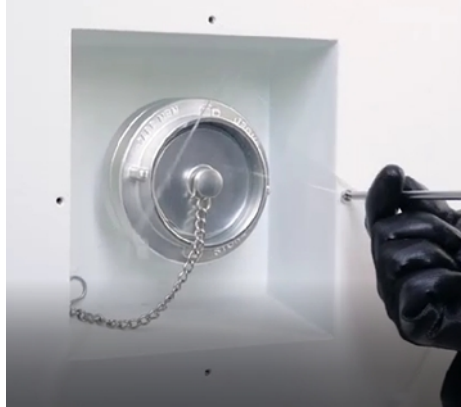
Figure 4-450 Remove the water inlet cover
