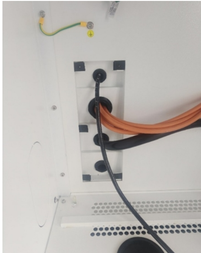
Figure4- 39 Panel ground cable installation
