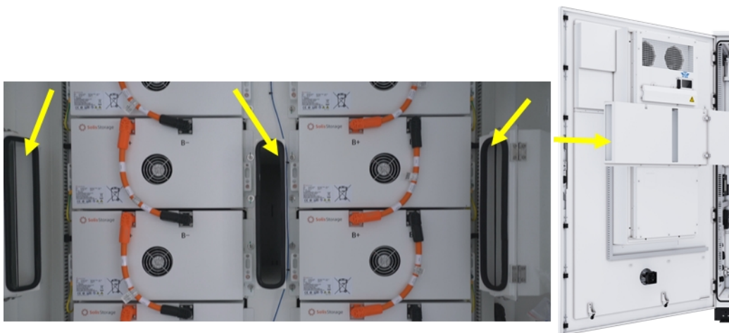
Figure 8-1 Check cable connection
