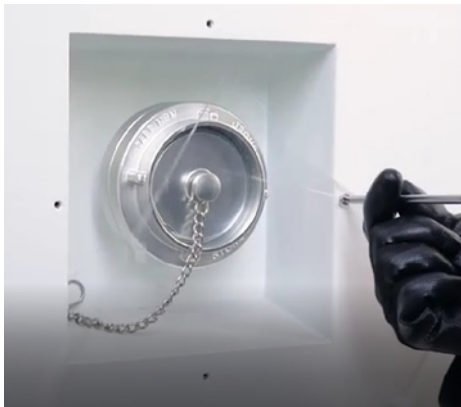
Figure 7-46 Remove the water inlet cover
