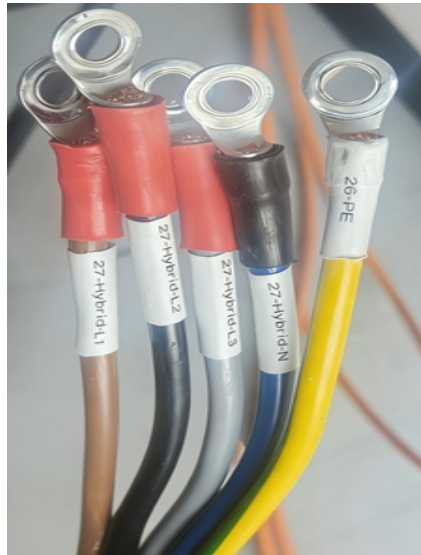
Figure 7- 17 Auxiliary power cable
