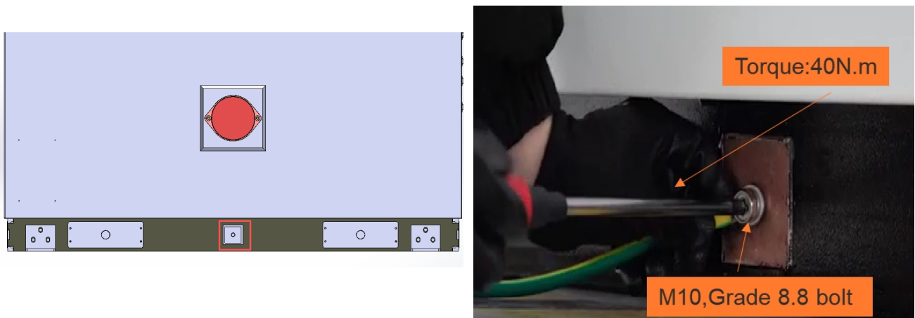
Figure 7-4 Cabinet ground connection
