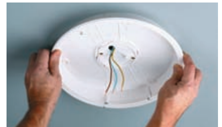
The insert attaches easily to the center plate with a simple twist
