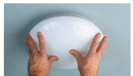
Finally, the diffuser is attached. Done!
