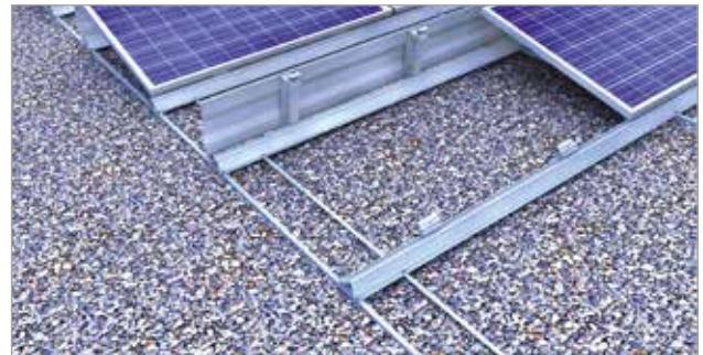
Gravel: South system I with cross rail
