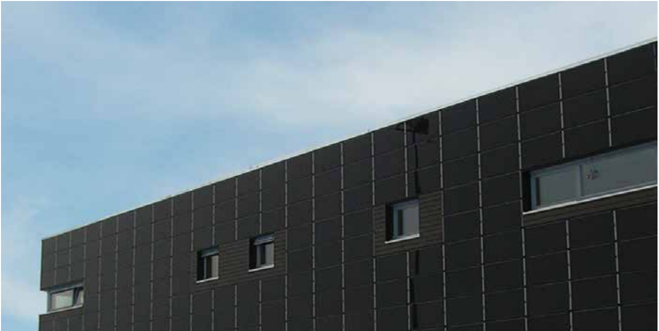
Using facade surfaces optimally
