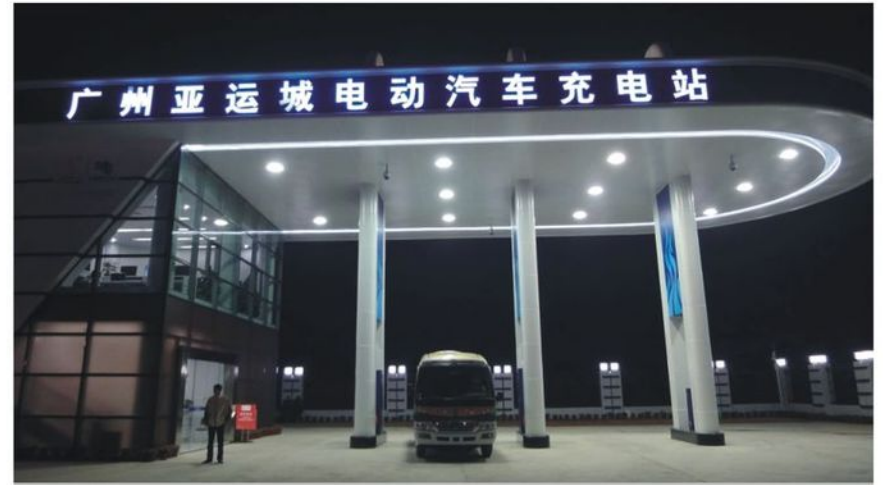
The Electric Vehicle Charging Station of Guangzhou Asian Games
