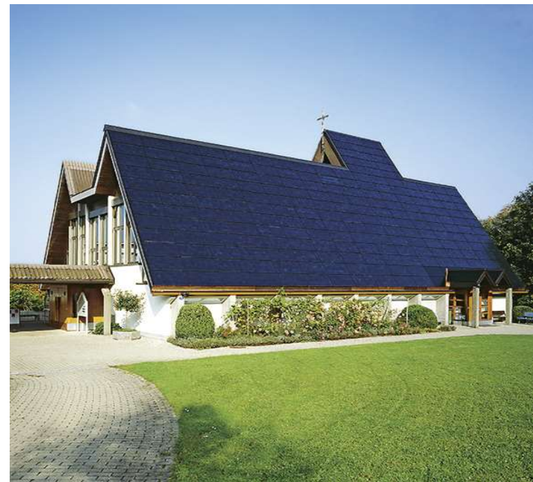
Complete roof modern church Switzerland
