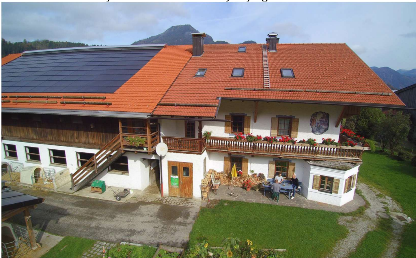
Stockfarm Germany: Air extraction for hay drying
