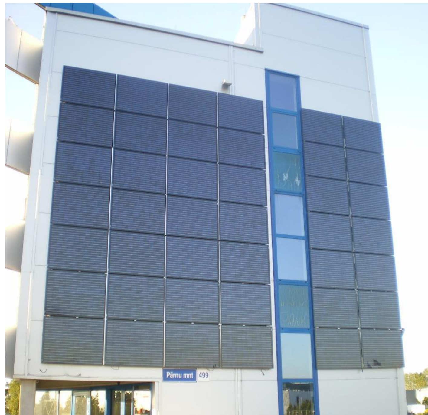
Baltic Disk integrated facade, 12 kW, Estonia
