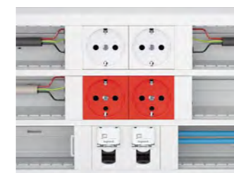
Example of installation: One current type per compartment
