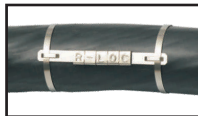
Marker Tags Installed on Power Cable
