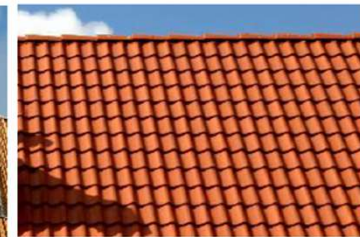
Roof with ceramic tiles
